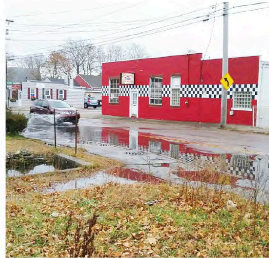
Sunny day flooding in Warren, RI 46
